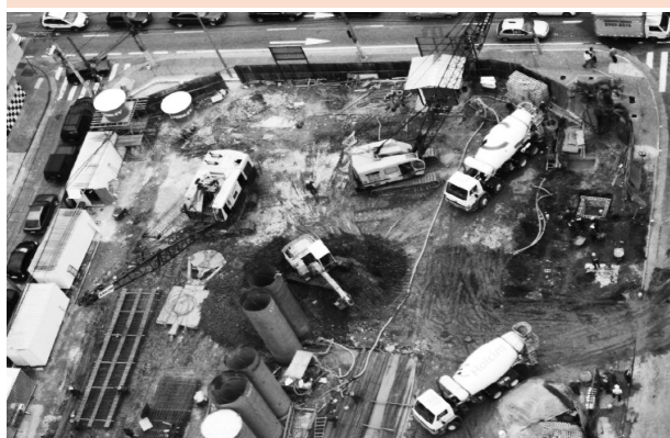
Figure 3: General view of the construction site
