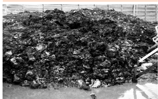
Figure 1: View of the excavated soil using bentonite slurry
