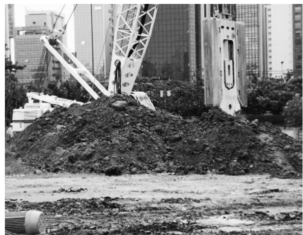
Figure 2: View of the excavated soil using polymeric slurry
