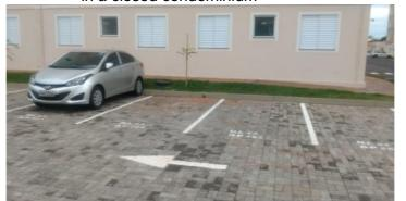
Figure 7 - Permeable pavement in the form of interlocked concrete used in a closed condominium
